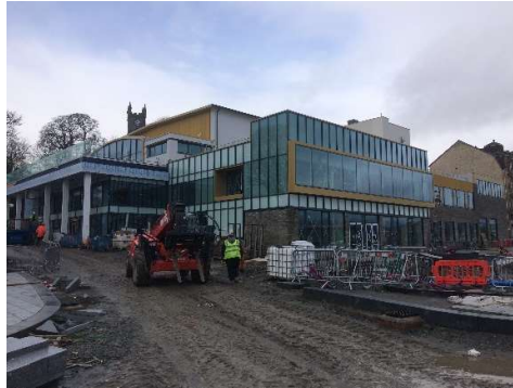
South and East Elevations
